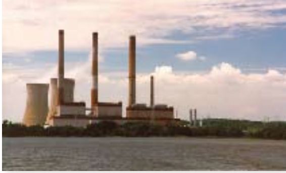
Left: Pepco power plant in Benedict, Maryland [www.aceinc_umces.org]. Below: Pepco customers in the D.C. area [www.sprol.com].
