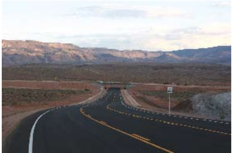
River Road, a feeder road of Southern Parkway leading the new St. George City airport in Utah.
